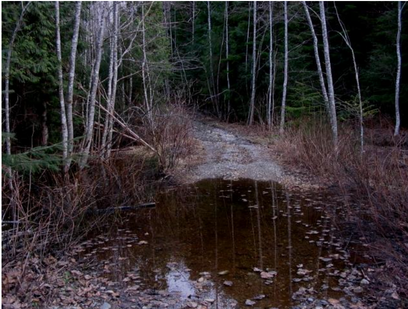
Stream crossing without bridging – Scully Creek area.
