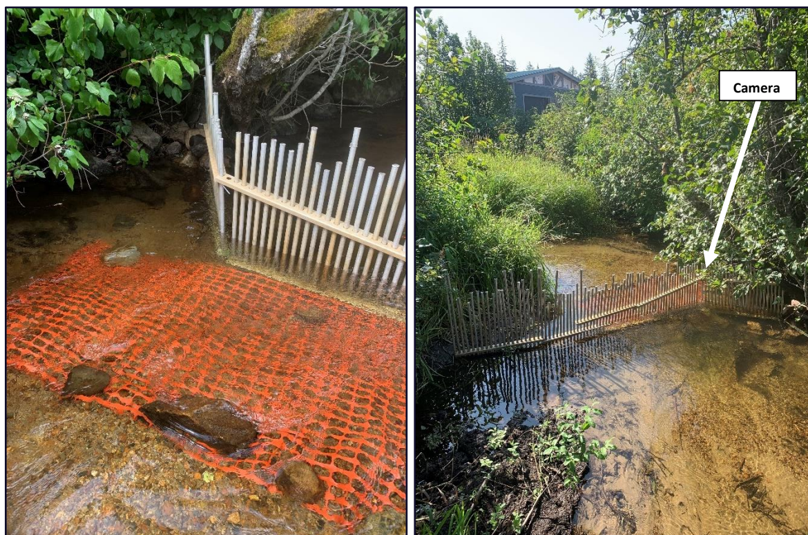
Figure 3. Upstream snow fencing (left) and completed fence with camera installed (right).
